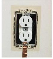
Turn off power to outlet, remove faceplate cover, remove bottom screw holding outlet to conduit box, start the 1/2 wide adhesive backed copper foil tape as shown, place screw through copper, replace ac face plate cover, restore power.
