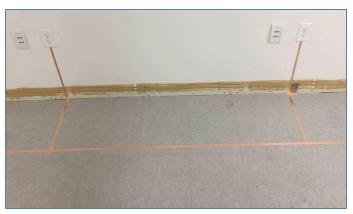
Method one: A Copper strip is placed over the ground strips coming down from the outlet (or steel structural support columns) and is run the full length of one wall. When the tiles are placed over the copper strip running parallel with the wall the entire structure becomes grounded. ElectraLock has excellent tile to tile conductivity due to the full surface conductive backing.
