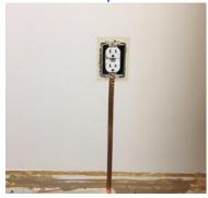
Run ground foil down wall and onto substrate about a foot or 2. Hint: Use an L square to keep it parallel or it may bother you long term! It's fine to attach to multiple outlets. This same method may be used to attach to steel structural support columns as well.
